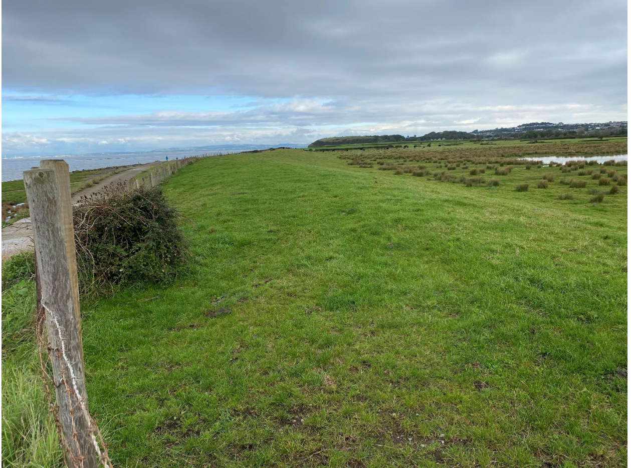
Figure 4 – Photograph looking north along existing earth bund. Taken on 9 th October 2024 during site walkover.
