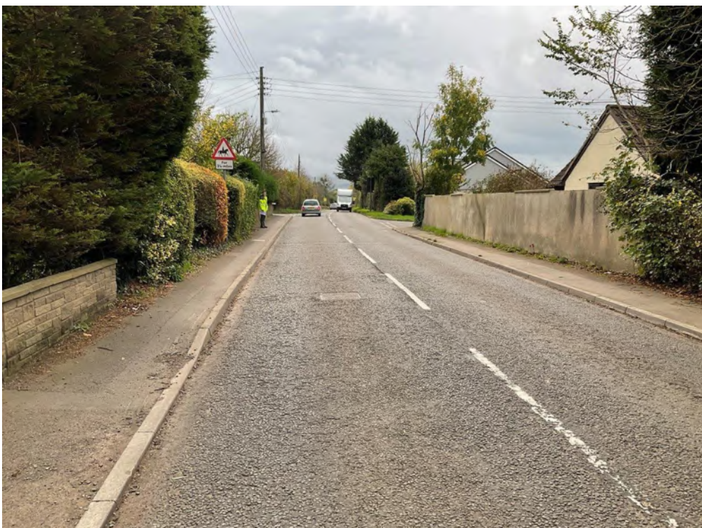
6.2 General view looking south on Brinsea Road
