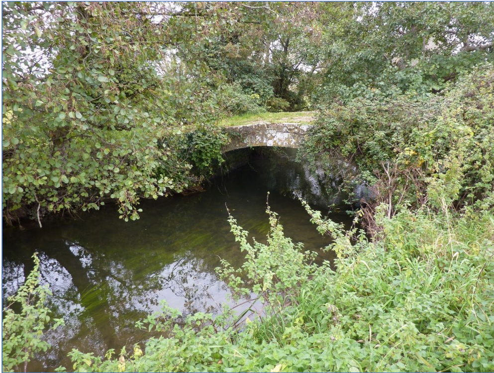
Figure 14 Collins Bridge, looking in direction of PDA (not visible)
