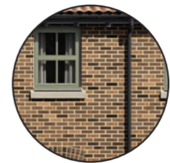
Rainwater goods black finish, with mix of black and white fascia and barge boards
