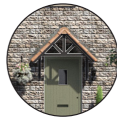
More limited use of brickwork compared to render and recon stone. Mix of mono-pitch and cottage style entrance canopies
