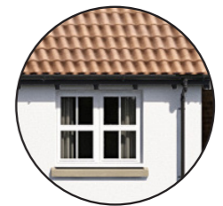
Rainwater goods black finish, with mix of black and white fascia and barge boards
