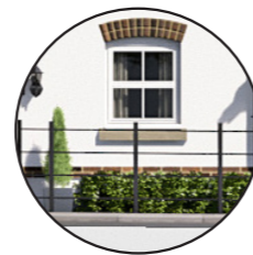
Painted black metal estate railings on key frontages and corners with low shrub planting to define defensible space
