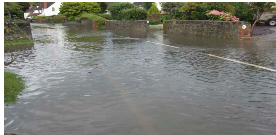
Surface Water Flooding at Elm Tree Road in Locking (2012)
