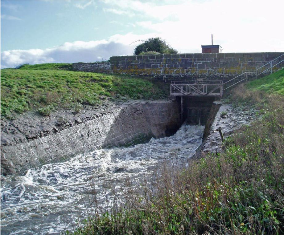
**Image 11.** It Shows Sampson's Sluice, where the Oldbridge River meets the flood defences along the coast. Sluices and flaps like these ensure a continuous line of protection along the coast.
