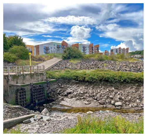
**Image 12.** This is a tidal flap at Portishead's end of the Portbury Ditch. The flap lets water out when the tide is low and holds the tide back when the sea rises against the flap.
