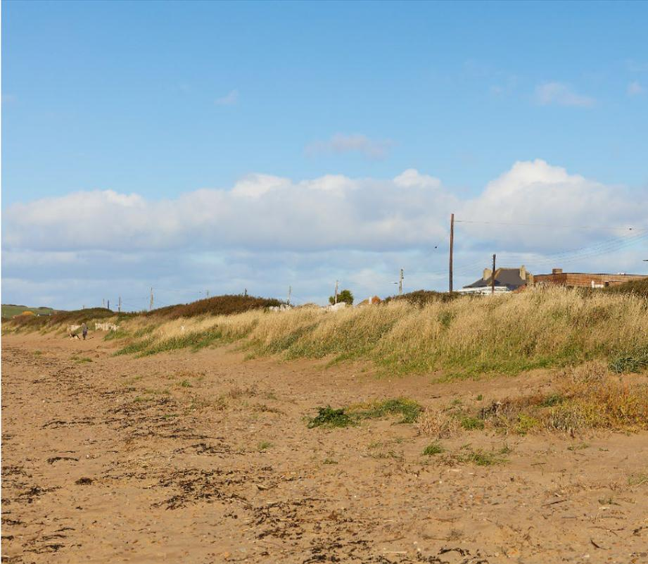
**Image 9.** The dunes at Sand Bay are an integral part of the flood defences that protect properties nearby. They are artificial - in 1983/84, over 600,000 tonnes of sand were dredged from the Severn Estuary and pumped onto the beach, raising it by approximately three metres at the sea wall.
