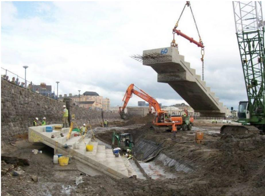
**Images 3 and 4.** At Weston-super-Mare, the Victorian sea walls have already had an upgrade. Concrete steps have been built in front of the old walls to prevent waves from damaging the bottom of the wall. New walls were also constructed behind the promenade to protect properties from large waves that overtop the old walls. These were also designed so that they can be raised when needed in the future due to sea level rise.
