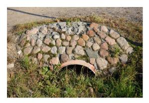
**Image 3**. A blocked culvert no longer allowing water to flow through it.
