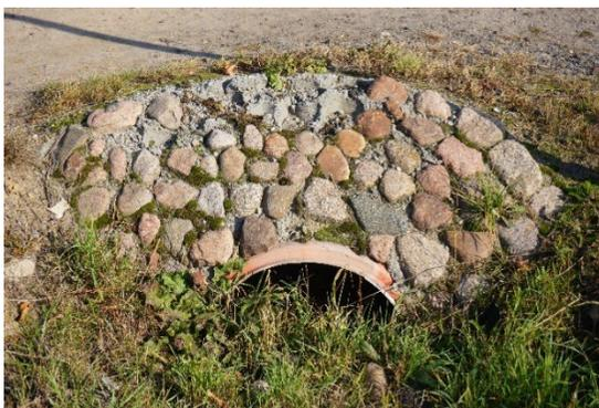
**Image 3.** A blocked culvert no longer allowing water to flow through it.
