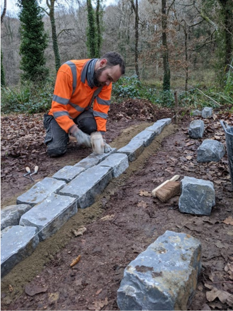
Images 21 and 22. Installation of the stone track drainage features
