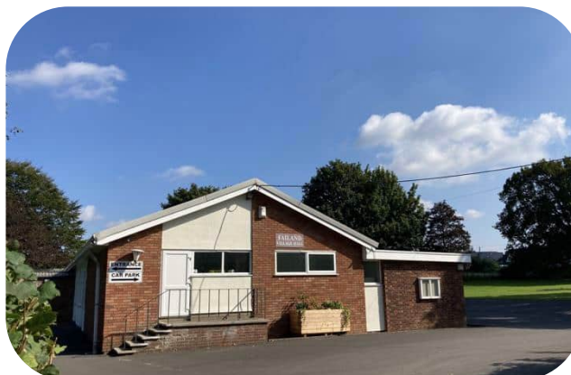
Figure 9 - Failand Village Hall
