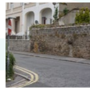
Stone boundary walls
