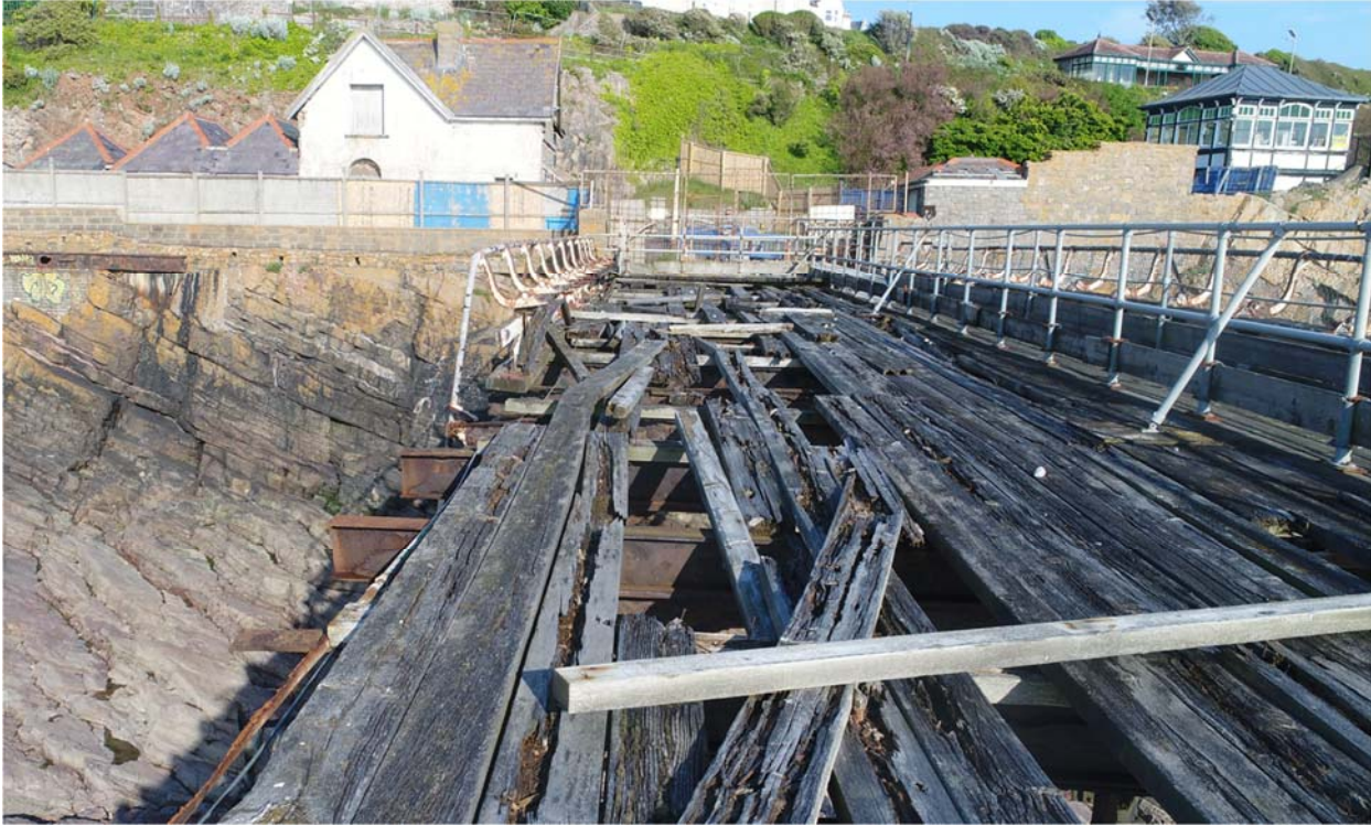
Pier Master's Cottage from the Pier 24 May 2023
