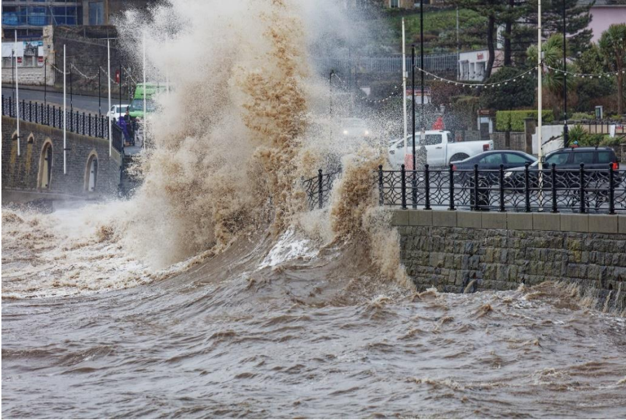
Images 1 and 2. The Victorian sea walls at Clevedon protect residents from flooding when there is a combination of high tides and stormy weather.
