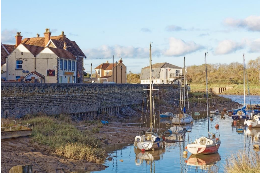
Images 5 and 6. At Pill, the walls and flood gates prevent high tides and storm surges that flow up the River Avon from flooding nearby properties.
