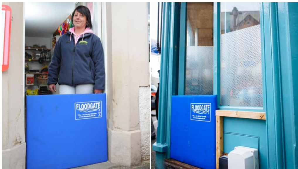
Figures 22 and 23: Examples of property level flood resilience measures.
