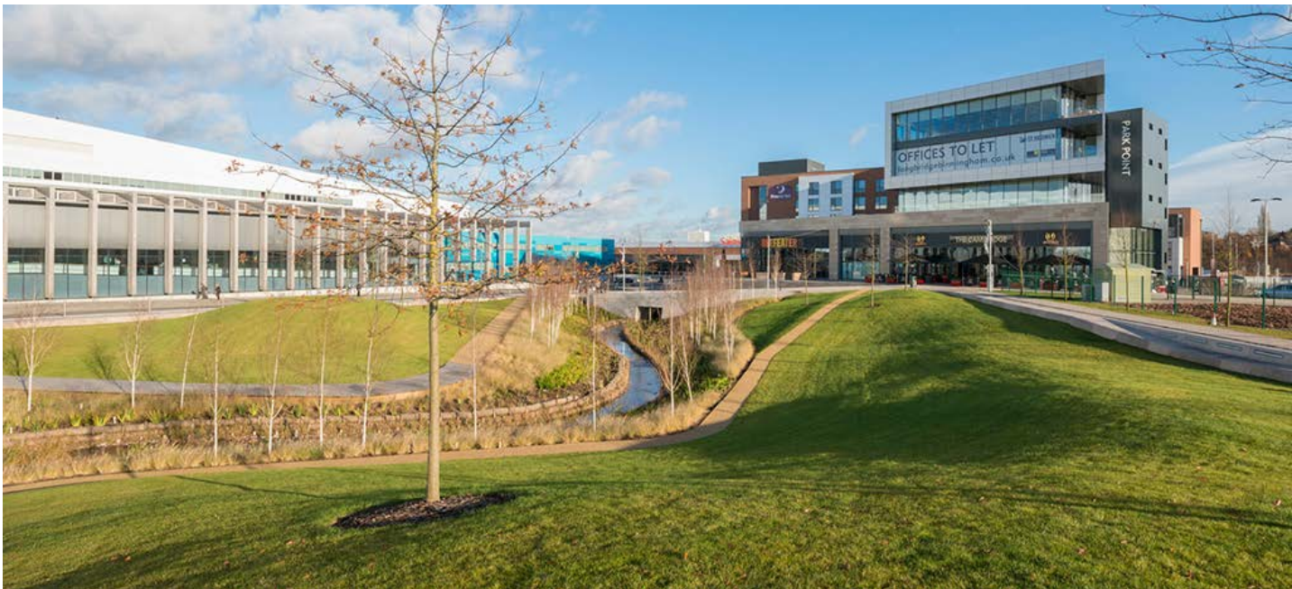
Figure 18: The redevelopment at Longbridge integrates the River Rea and ensures buildings are resilient to flooding.
