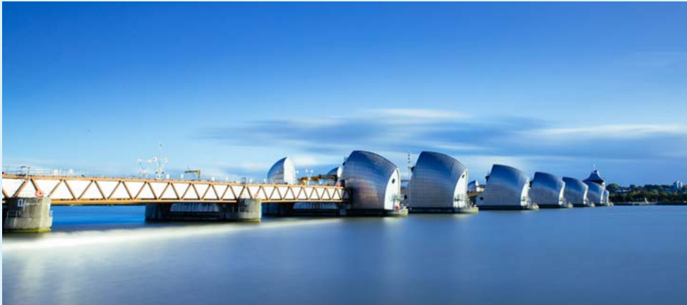
Figure 12: The Thames Barrier, London.
