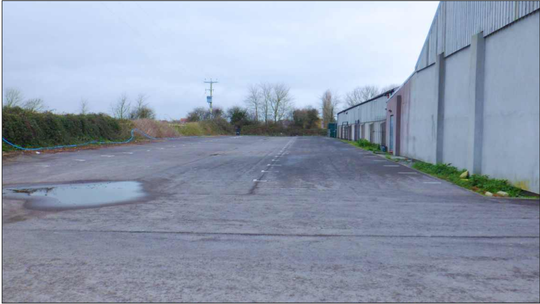
Plate 7: View to the east showing Plot 5 which comprises a car parking area to the north of the industrial units on the north side of Ebdon Road
