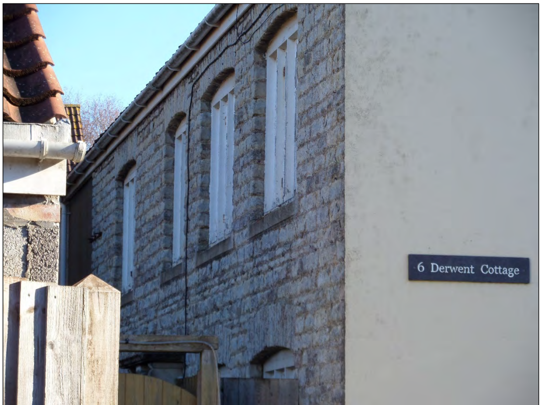
Photo 2 Close-up showing stonework on northern elevation
