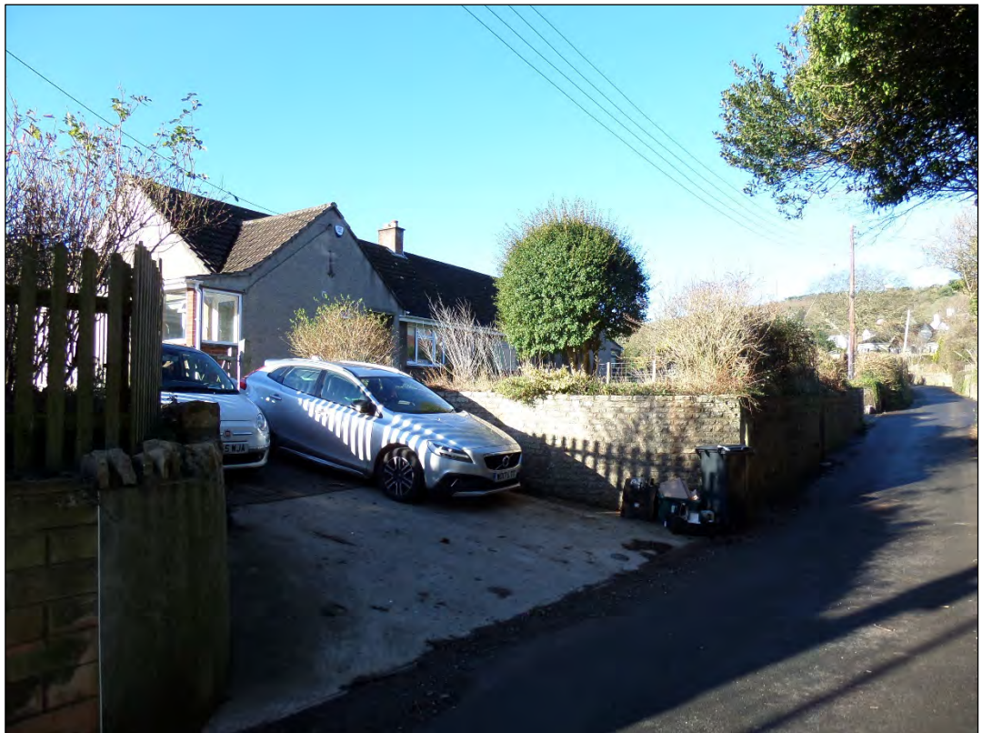
Photo 7 Driveway and façade of 1 Warren Lane
