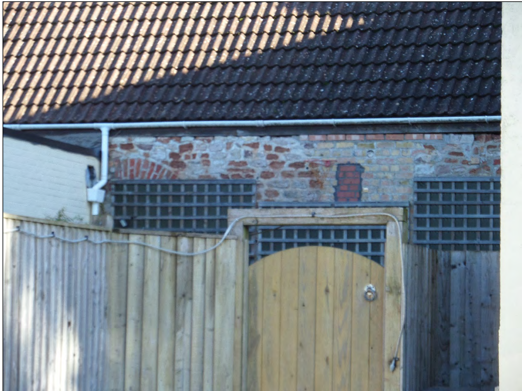
Photo 3 Close-up of stonework and brickwork of western elevation of adjacent outbuilding
