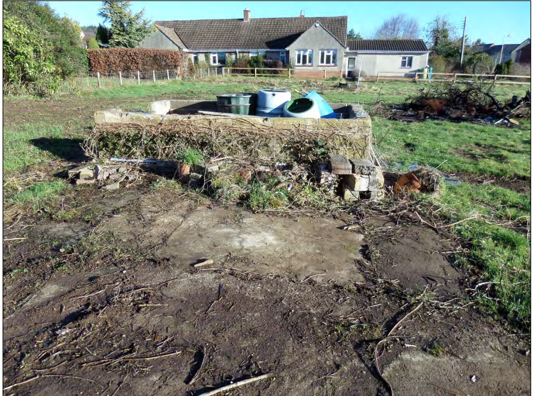
Photo 6 Hardstanding and walls of former greenhouse within western part of the Site
