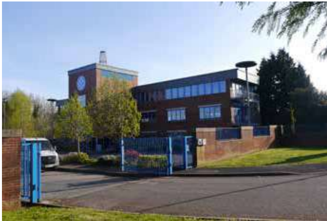
Office building - residential conversion underway
