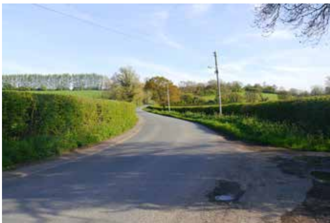
Road frontage to the sites looking south
