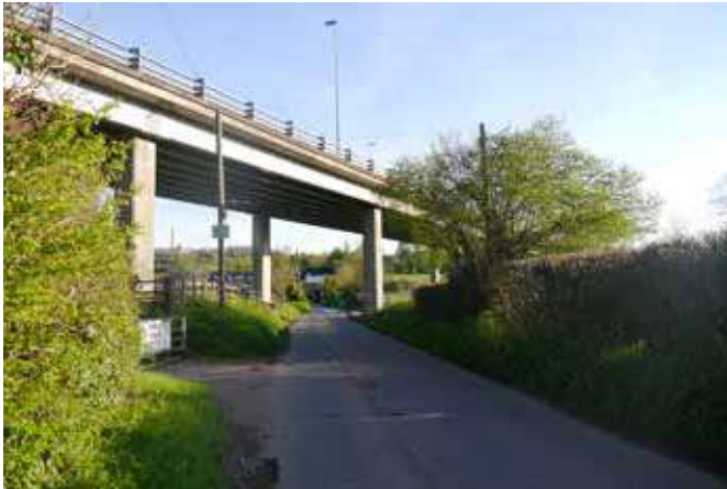
Site frontage to Yanley Lane
