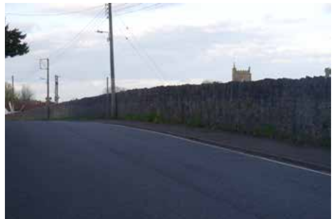
Site frontage on to Long Ashton Road
