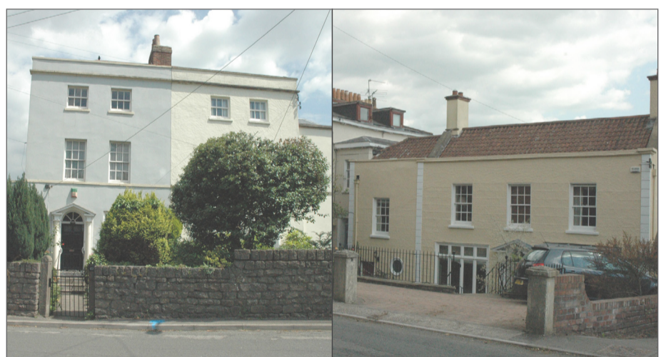
Figure 2.16: Local Examples - Render with parapets
