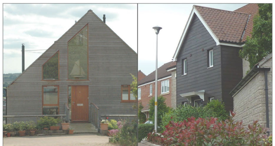
Figure 2.17: Local Examples - Timber cladding
