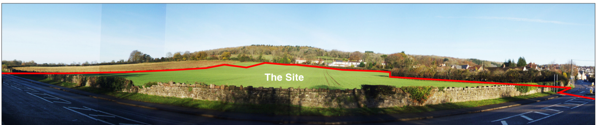
Figure 2.1: Panoramic View 01 from Weston Road looking north towards the site
