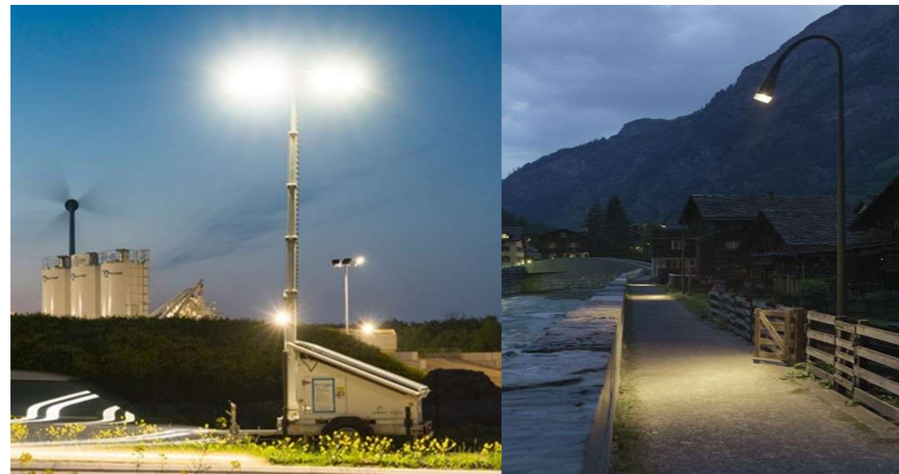
Figure 1 Comparison between high and low mounting scales. Image on the left shows large scale lighting column without any glare control and the image on the right shows a smaller column with controlled lighting distribution providing light to the path only
