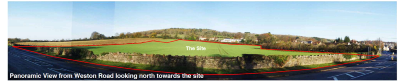
Figure 2.1.2 Street view of site boundary - Image courtesy of Nash Partnership.
