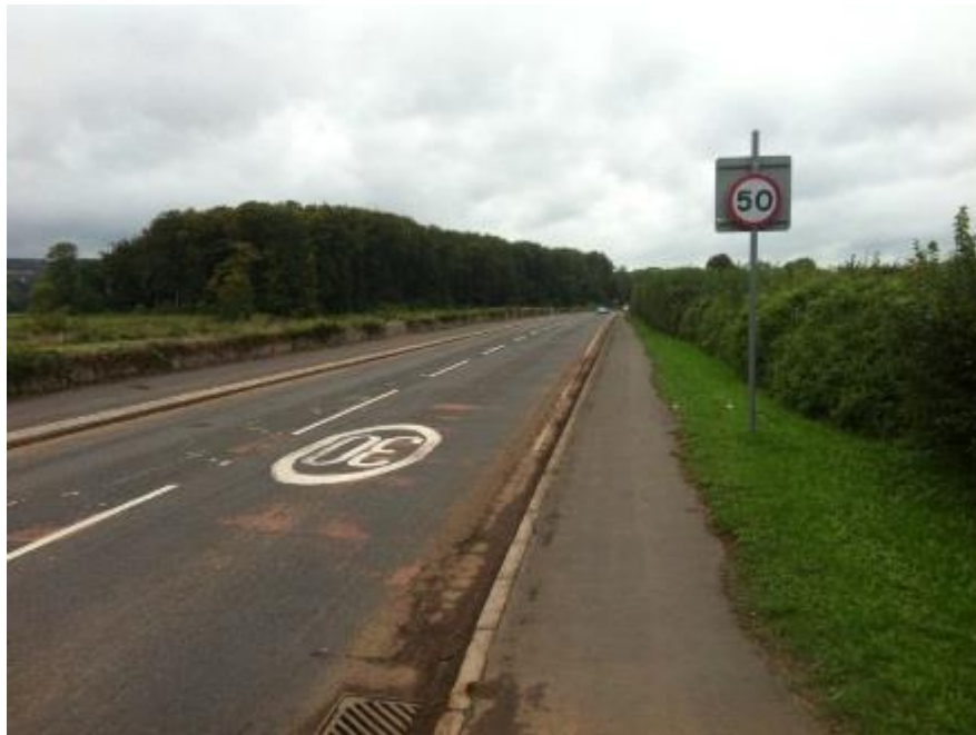
Photograph 2.1: Weston Road looking west along site frontage
