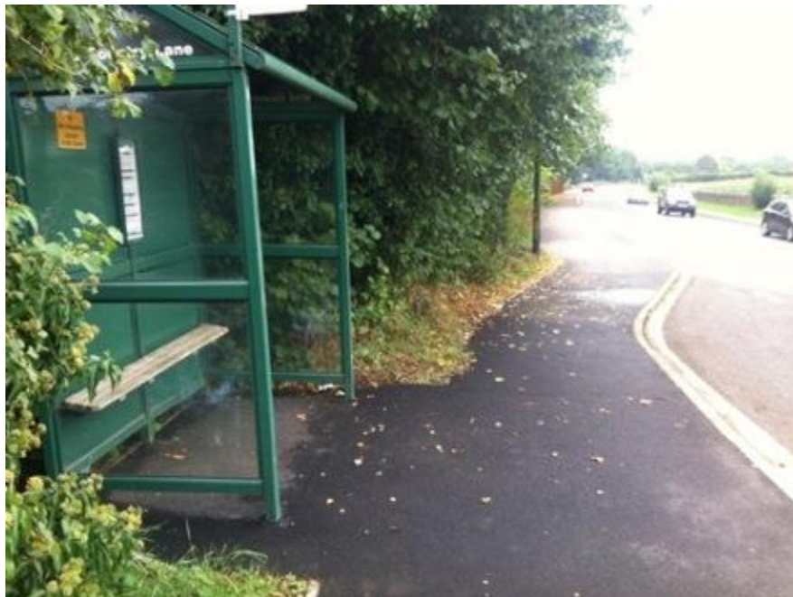
Photograph 4.3: Eastbound bus stop - Weston Road / Wild Country Lane
