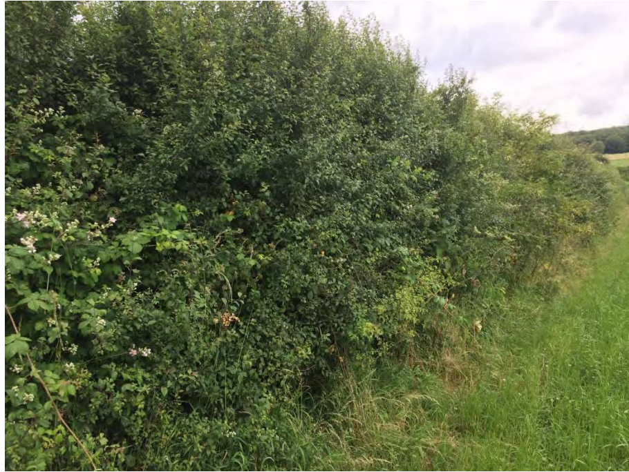
Photo 3: G6 hedgerow tree belt with remnant timber fencing and naturalised scrub / bramble cladding requiring selected thinning.
