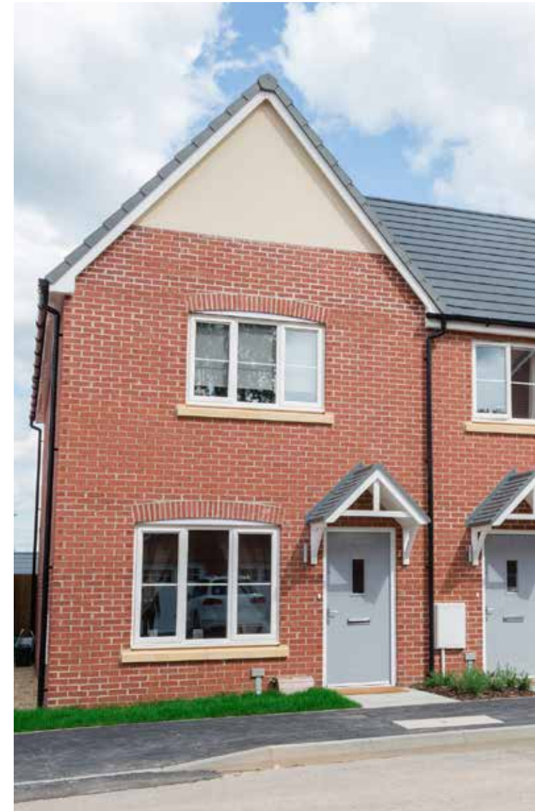
New build homes on Kestrel Road, Sandford. Photo by Alliance Homes
