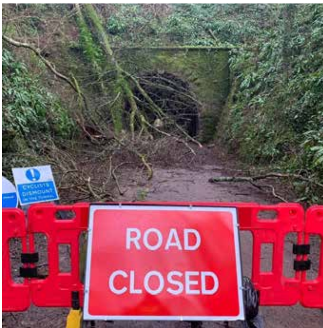
Figure 12: Photo of a fallen ash on a Public Right of Way
