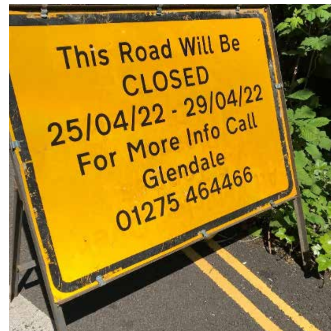
Figure 11: Photo of traffic management required for tree works on the highway
