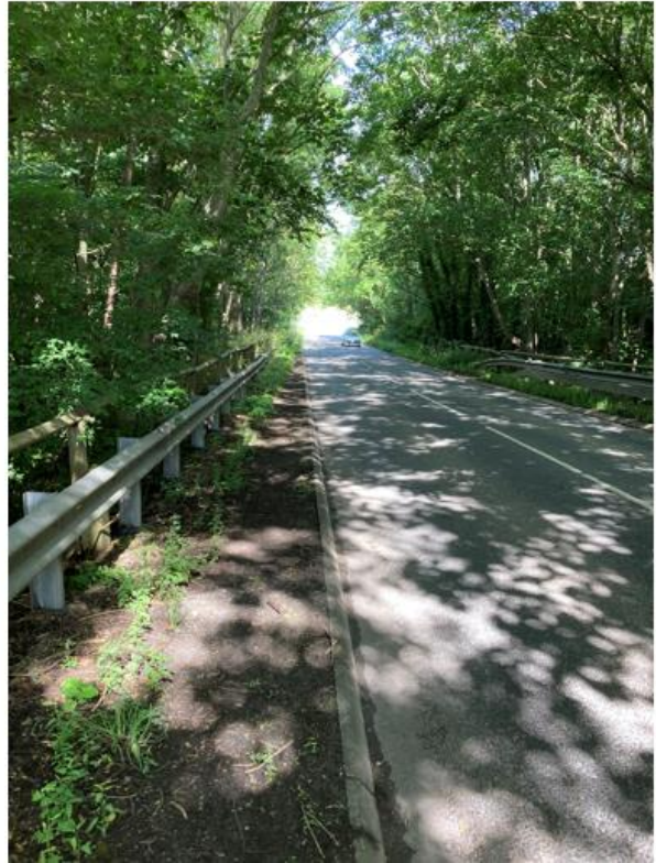
Wolvershill Road Bridge
