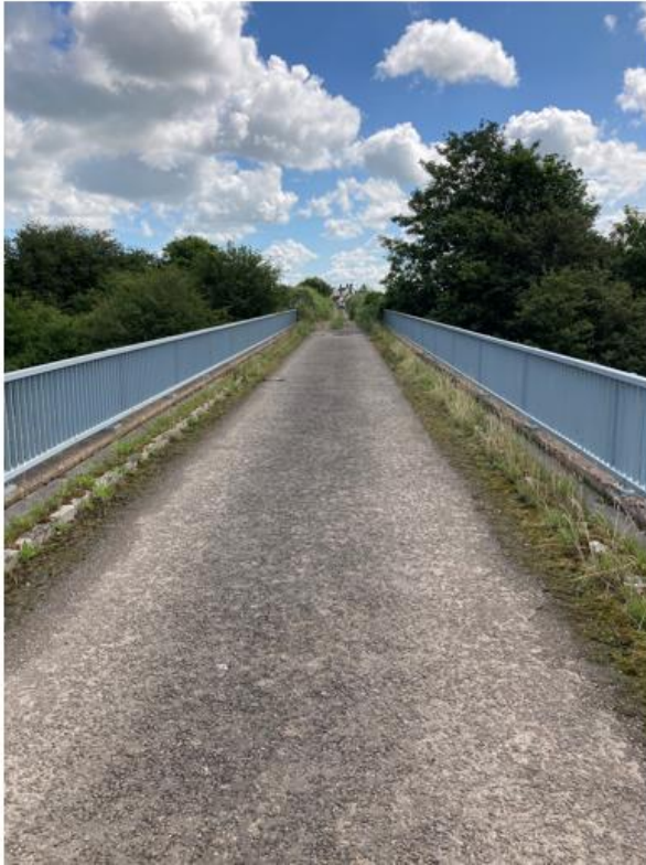
Existing Agricultural Bridge
