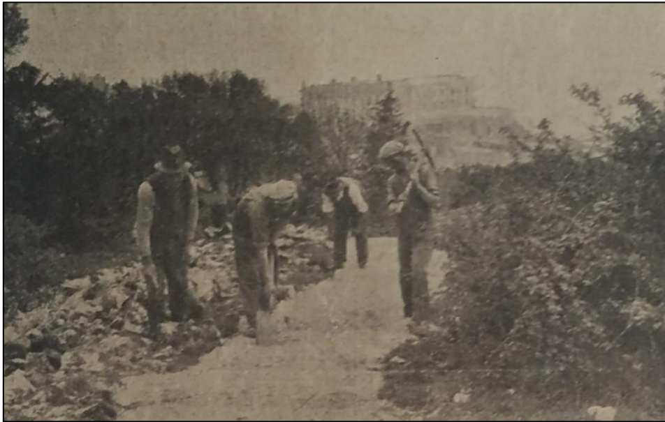
Figure 8: Workmen constructing path (Weston Mercury & Somersetshire Herald (1939))
