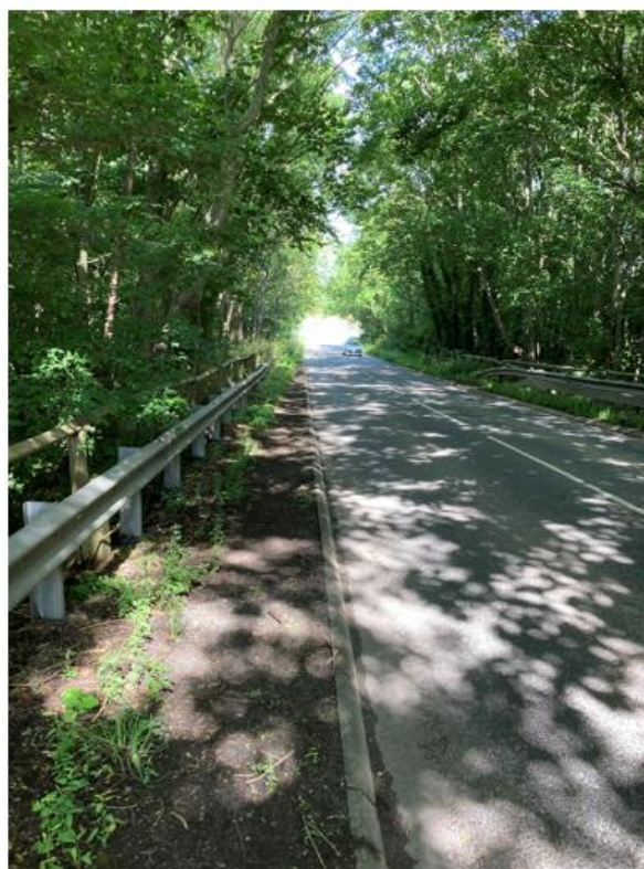
Wolvershill Road Bridge
