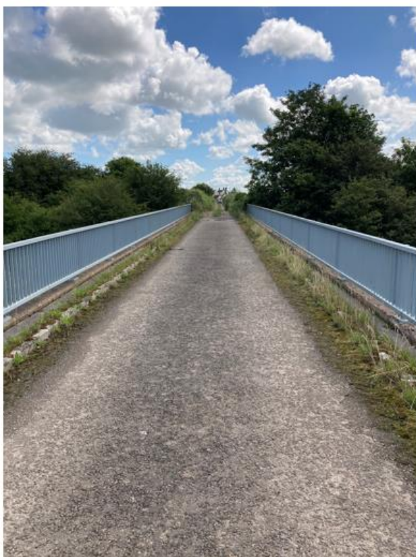
Existing Agricultural Bridge
