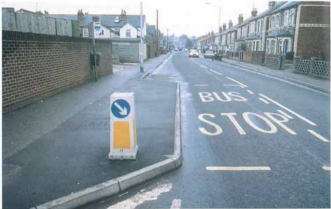
A bus boarder should be clearly visible at night. (Courtesy: Reading Transport Ltd).
