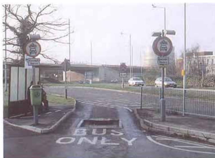
A bus gate with a physical obstruction to stop violations by cars.
