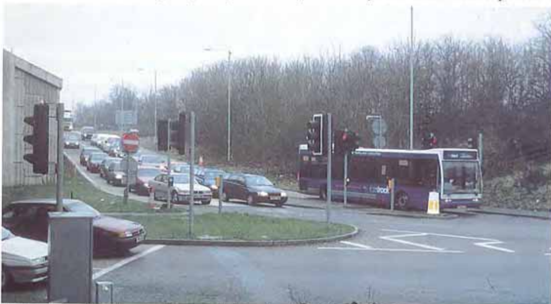
This bus lane allows buses onto a roundabout ahead of other traffic. (Courtesy: Reading Transport Ltd).
