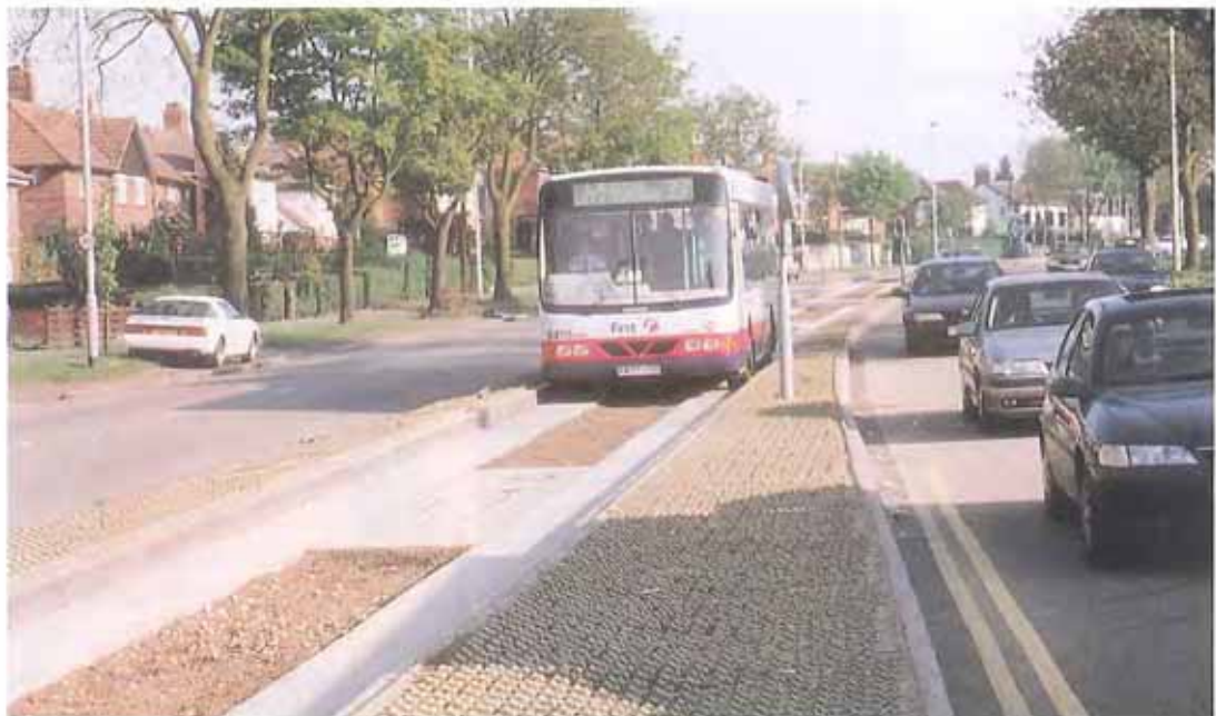
SuperBus in Leeds. The guideway in the central reservation acts as a self enforcing bus lane and gives priority at the next junction. (Courtesy: Leeds City Council and First Group).
