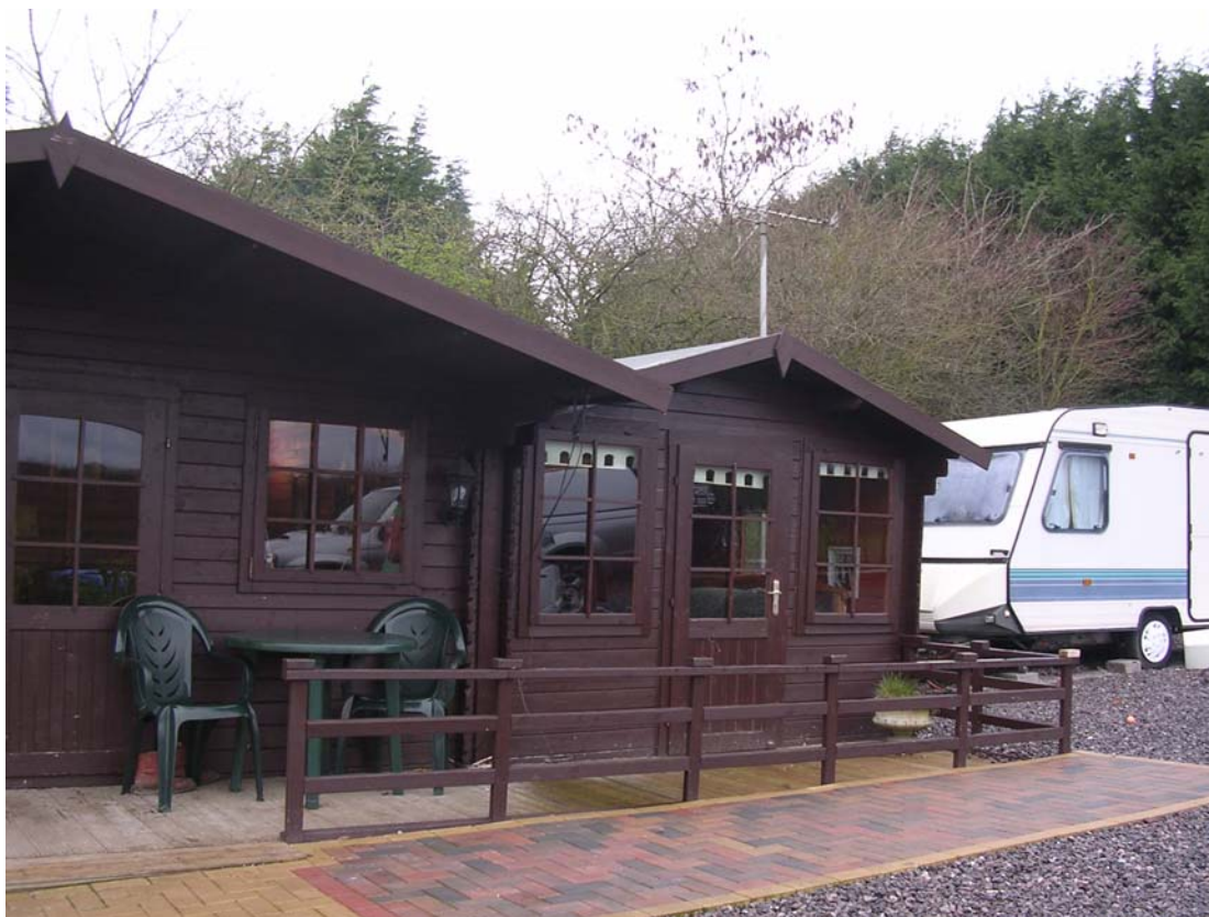
Plate 27: Utility buildings on private site in South Gloucestershire
