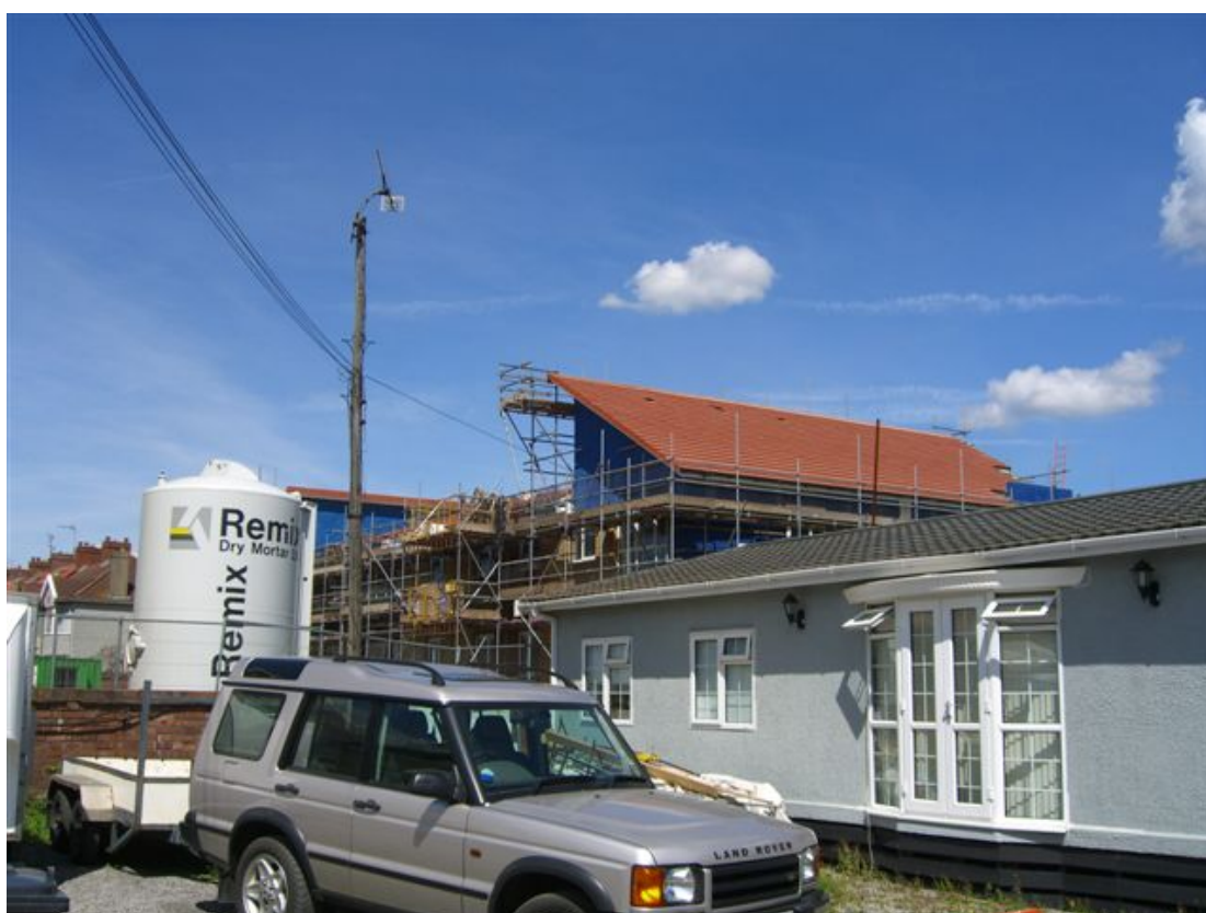
Plate 11: Showman’s Yard with mobile homes over-shadowed by adjoining building works
