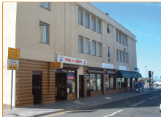
Photo No.2 – No 2a and 2b Oxford Street
