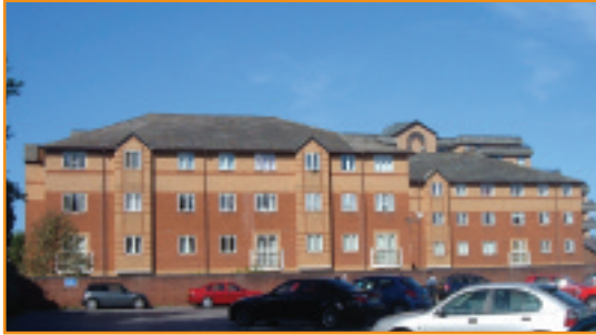
Photo No.5 – Residential properties facing Carlton Street car park
