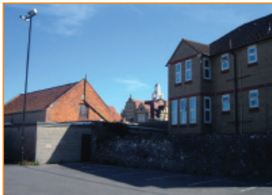
Photo No.3 – The NALGO building with its entrance from Carlton Street Car Park
