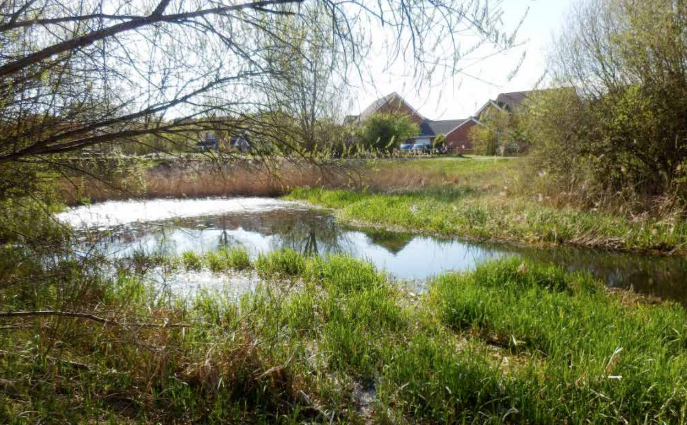
Portishead Wetland and Attenuation Pond (photograph from NSC)
