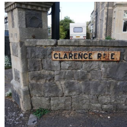
Stone wall and cast iron street sign
